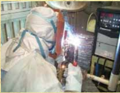
MIG・MAG welding
