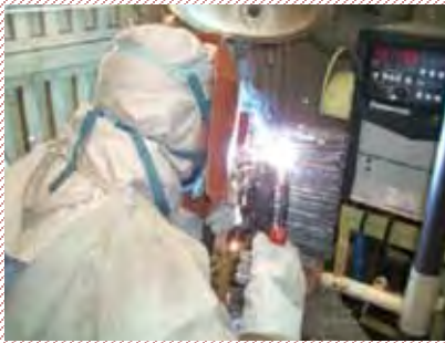
MIG・MAG welding
