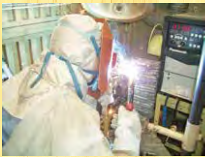
MIG・MAG welding
